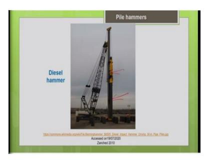
Let us see the picture of this diesel hammer you can see, this is a picture of the diesel hammer lifted by a crane. So, it is driving a steel pile, you can see this is a diesel hammer, this is a pile, it is lifted with the help of your crane.
